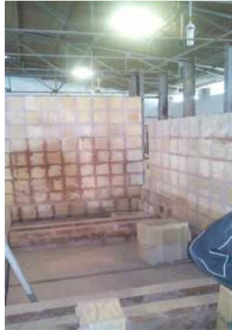
Historically, all the furnaces were lined by pressed, standard sized bricks in all the cases. So the wall thickness in all the furnaces was either 12-18 or 24 inches thick or even more, irrespective of its requirement. Anything less than 9" long was not available and hence they will use only this. Insulating materials like the Ceramic Fibre, the ULTRALITE, the Vermiculite got discovered in the last ten to twenty years.
