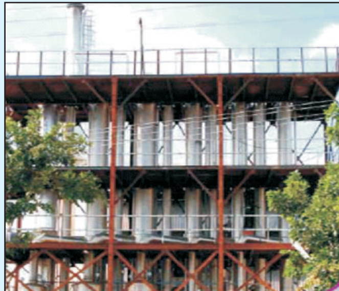
Fig. 10 : Machinery used in separation process
