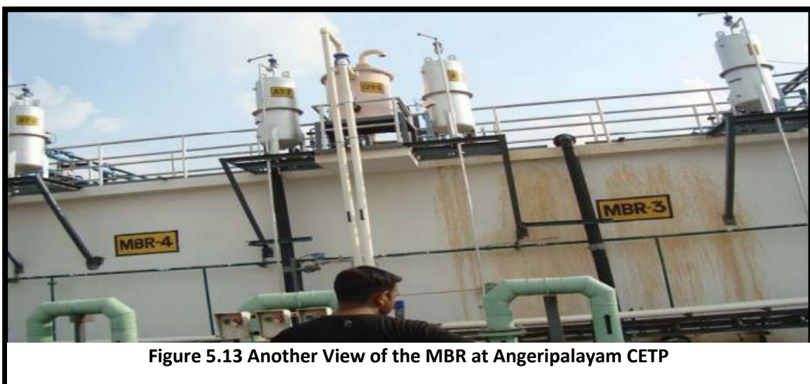
Figure 5.13 Another view of Membrane Bio Reactor installed at Angeripalayam (Tiripur, Tamilnadu) CETP
