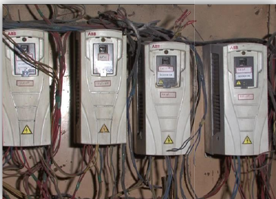
Installation of Invertors
