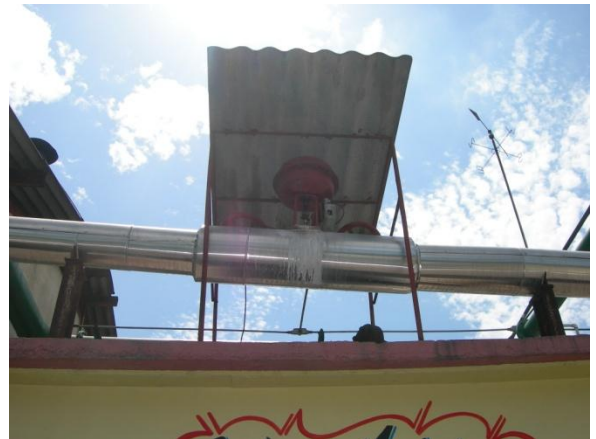
Figure 2. Insulation the steam distribution line
