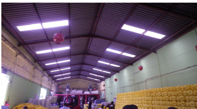
Production floor before and after installation of translucent sheets under RECP Implementation
