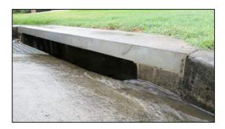
Side inlets type storm water drain with screen
