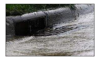
Side inlets type storm water drain
